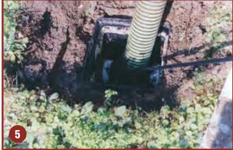
Be sure to inspect all connecting junction box locations (level, repair and adjust distribution flow), then jet junction boxes and drop boxes (to achieve adequate flow and distribution of materials during remediation, and following the treatment process).
