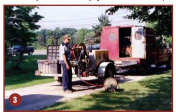
Following pumping and cleaning of all system tanks, jet and vacuum all absorption field lines.
