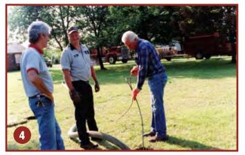
System jetting will remove trash, line deposits, and bio films, and allow adequate distribution of the bio-remediation treatment to the absorption system.
