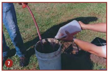
Blend each *PRO-PUMP* material with tap water prior to addition to the system.
