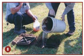
Following dilution with tap water add the *PRO-PUMP* formulations directly to the absorption systems via the systems junction box.
